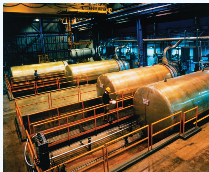
Figure 2.9.2: A Portion of a Plant for Separating Uranium Isotopes by Effusion of \text{UF}_6 . The large cylindrical objects (note the human for scale) are so-called diffuser (actually effuser) units, in which gaseous \text{UF}_6 is pumped through a porous barrier to partially separate the isotopes. The \text{UF}_6 must be passed through multiple units to become substantially enriched in ^{235}\text{U} .
